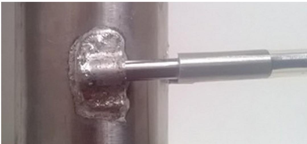
What are the advantages of this method – ease of installation and removal of the sensor, absolute tightness of the connection, no need to drill a hole and install a fitting.
